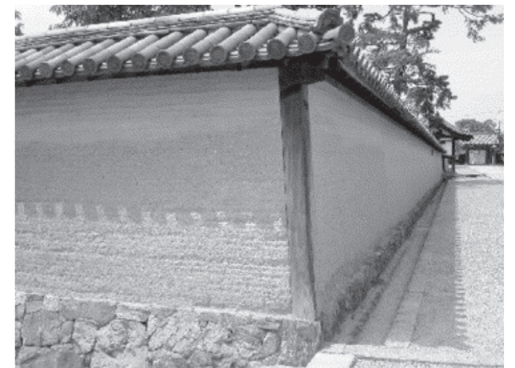
Figure 11. Horyuji Temple, Japan. At least 1300 years old rammed earth structure. Standing the test of time. Photo: D. Henman
