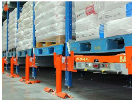
Figure 3.7: High-density deep-lane storage racking infrastructure optimized for autonomous radio-controlled pallet shuttle platforms (SSTC-storage, 2026)
