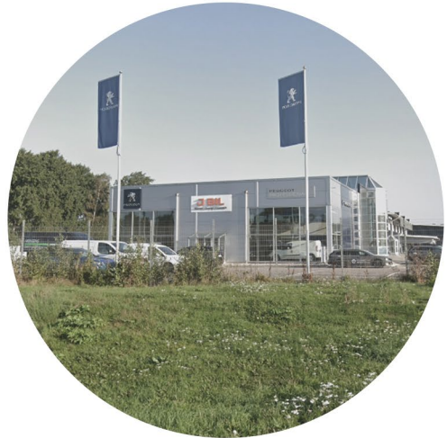
North: Equipment Rental Agency
