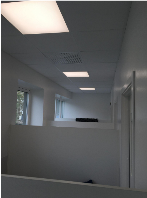
Figure 5. The semi walls between the boxes.
