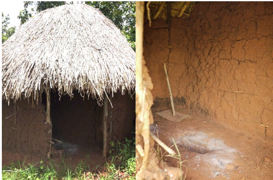
Figure 11. To the left is the small cottage where the toilet is located. For reference it is too small for anyone but children to stand upright in. To the right is the inside of the toilet cottage. Leaned on the back wall is the stick with a metal sheet on which is put on top of the hole to prevent smell.
