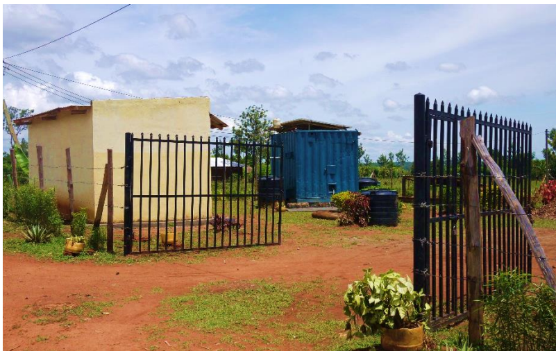
Figure 12 The area where the Kudura system is located. The blue container being the Kudura system itself and the white building being designated for future businesses.
