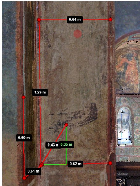
Figure 1: Measurements on the wall, screenshot from GRIDHs portal
