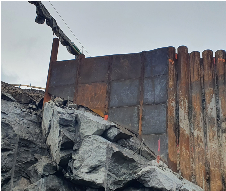
Figure 2.6: Sparse wall or "soldier pile wall", from the studied site.
