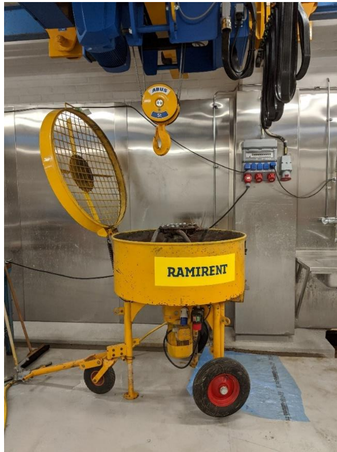
Figure A.5 Mixing of concrete batch on casting day.
