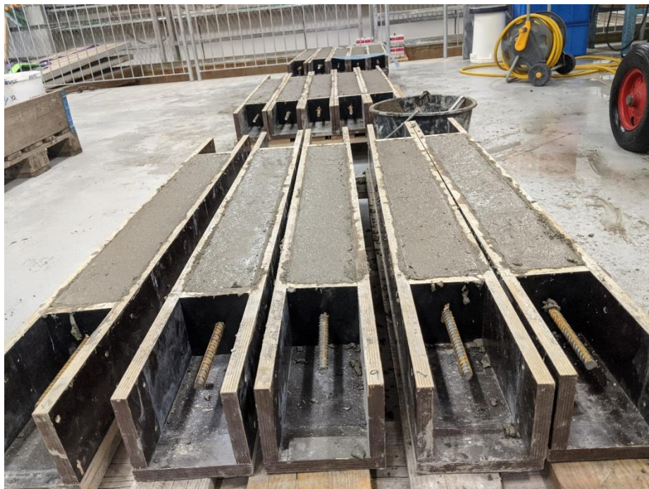
Figure A.6 Casting of the reinforced concrete prisms.
