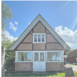
Surrounding residential buildings.
