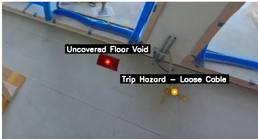
Figure B.2: Correctly identified hazard plus a false assumption = Overshot Positive AI-generated output.
