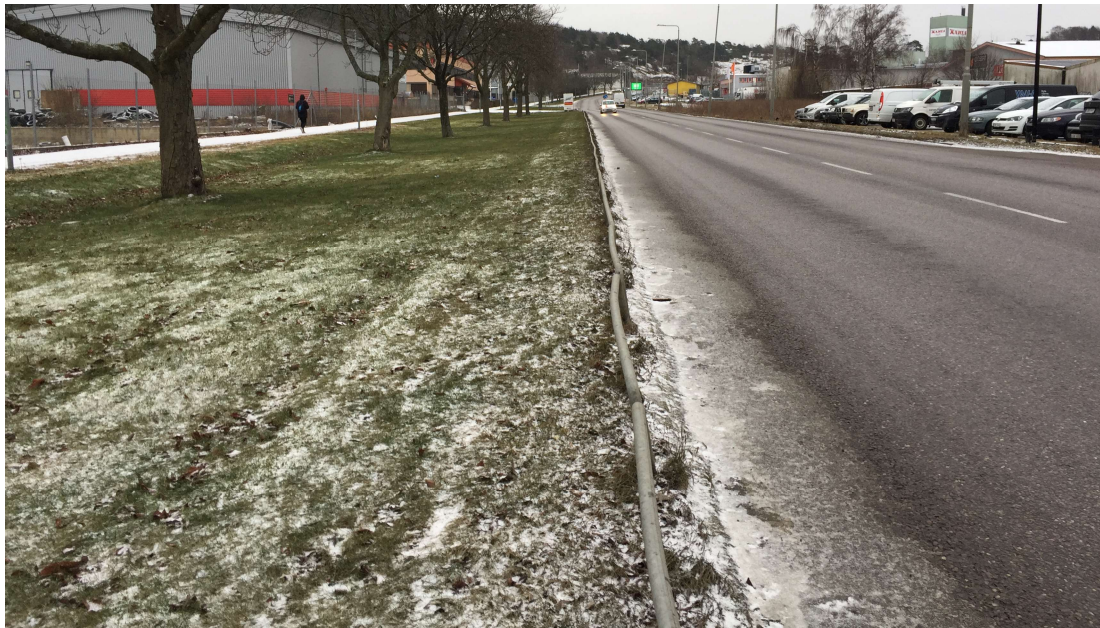
Figure A.3 Along a larger road within an industrial area in Dag Hammarskjöldsleden. Curb stones prevented the runoff from the traffic surface from draining to the possible ditch at left side of picture. (Photo by authors.)
