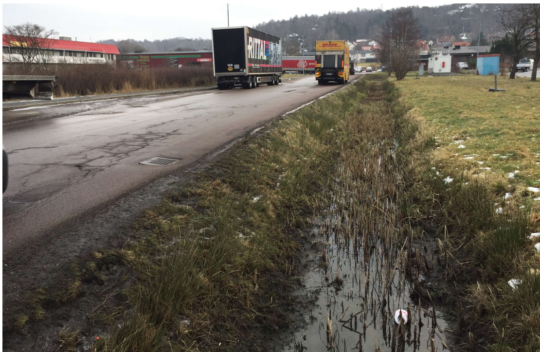
Figure A.2 Ditch in an industrial area in Lillhagen. The traffic-related stormwater not led to the pipe network through the storm drain, was drained to the ditch. (Photo by authors.)
