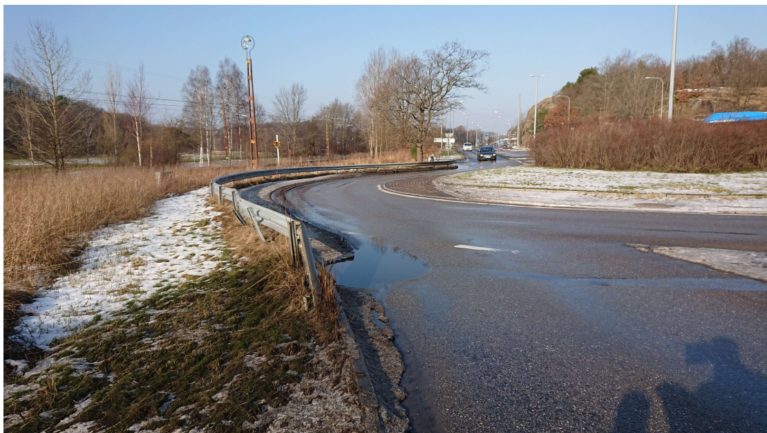
Figure A.6 Roundabout in Lillhagen, within the land-use nature, where curb stones prevented the stormwater from the road surface from being drained to the nearby green area. (Photo by authors.)
