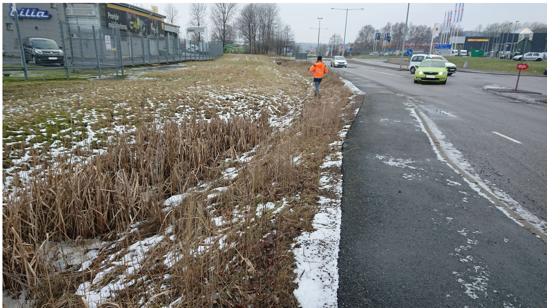
Figure A.8 The sidewalk prevented the traffic-related stormwater to reach the nearby ditch in Lillhagen. (Photo by authors.)
