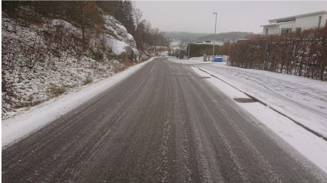
Figure A.7 In some areas in Lillhagen, the inclination of the roads tilted towards the sidewalk and the storm drains. Instead, the traffic-related stormwater could have been led to the ditch by using a super-elevated inclination tilting against the ditch on the left side. (Photo by authors.)
