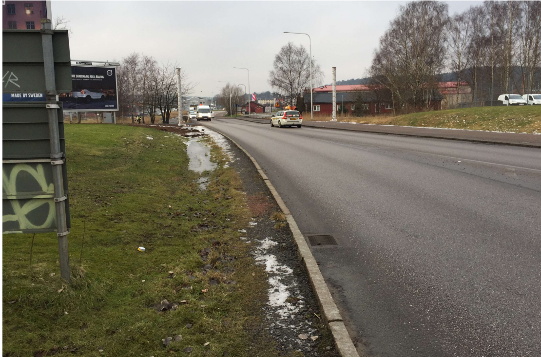
Figure A.5 Along a larger road in Lillhagen. Curb stones prevented the traffic-related stormwater from being drained to the green area. Instead, the water was led to the storm drain. (Photo by authors.)
