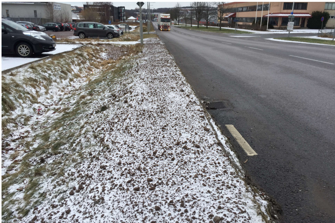
Figure A.4 Ditch along a larger road within an industrial area in Dag Hammarskjöldsleden. Curb stones prevented the runoff from the traffic surface from draining to the existing ditches at left side of picture. (Photo by authors.)
