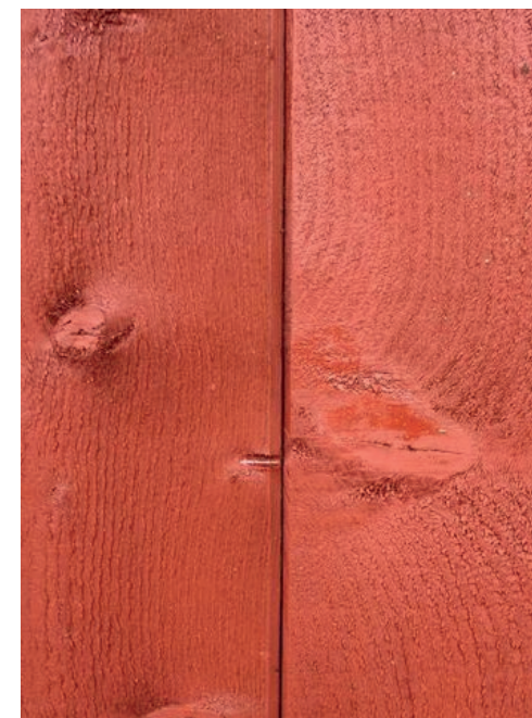
Exterior Panel treated with red pine tar
