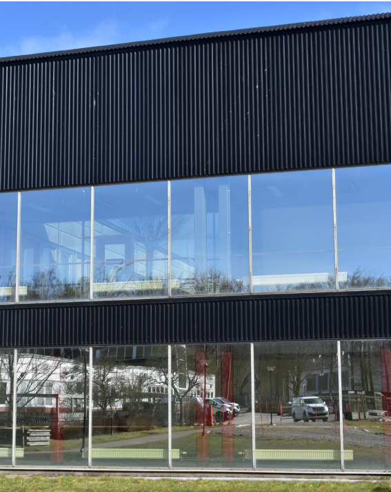
Corrugated metal facade with a band of glass. This is seen in the building north of the site where the new extension will connect.
