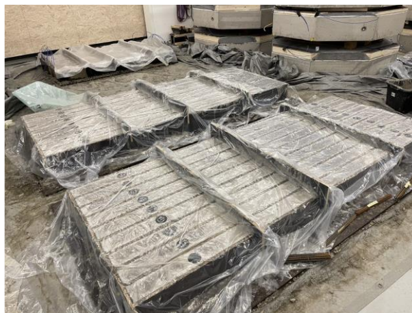
Figure 6.7 An illustration showing the covered concrete.
