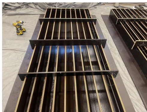
Figure A.1 Finalized mould with the overlaying support drilled on top.
