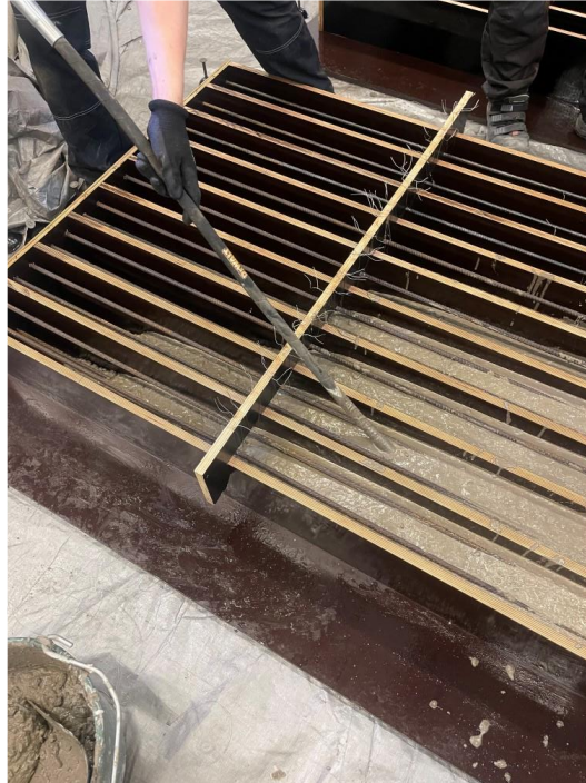
Figure 6.5 The vibrators that mixed the concrete in the forms.
