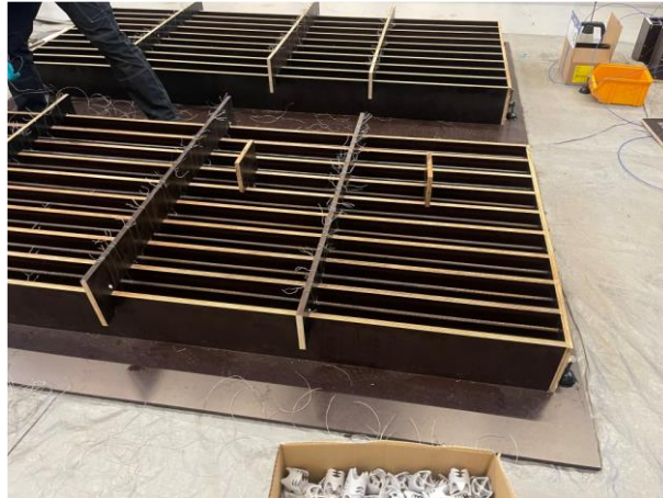
Figure 6.3 An illustration showcasing how the reinforcement was hung up with steel wires to the overlaying support.
