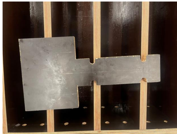
Figure 6.2 An illustration showing the T-section used to get an accurate concrete cover.
