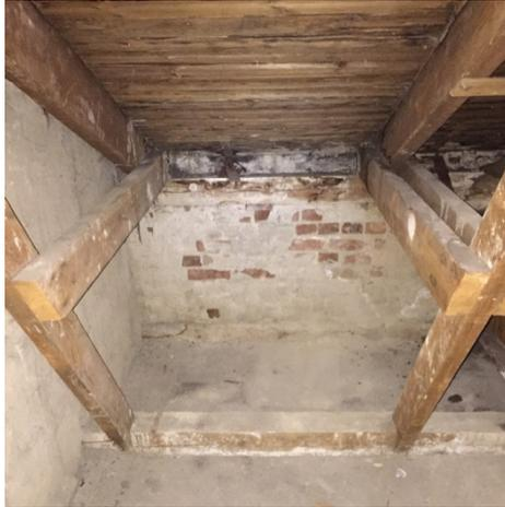
*Figure 5.9 Design of roof trusses and connection of roof and exterior wall. Notice the brick wall.*
