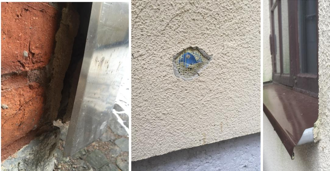
*Figure 5.2 Left: Added insulation layer behind covering steel plate in a corner. Middle: External stucco and fastening of the insulation visible through a damage. Right: Window ledge connection to the façade.*
