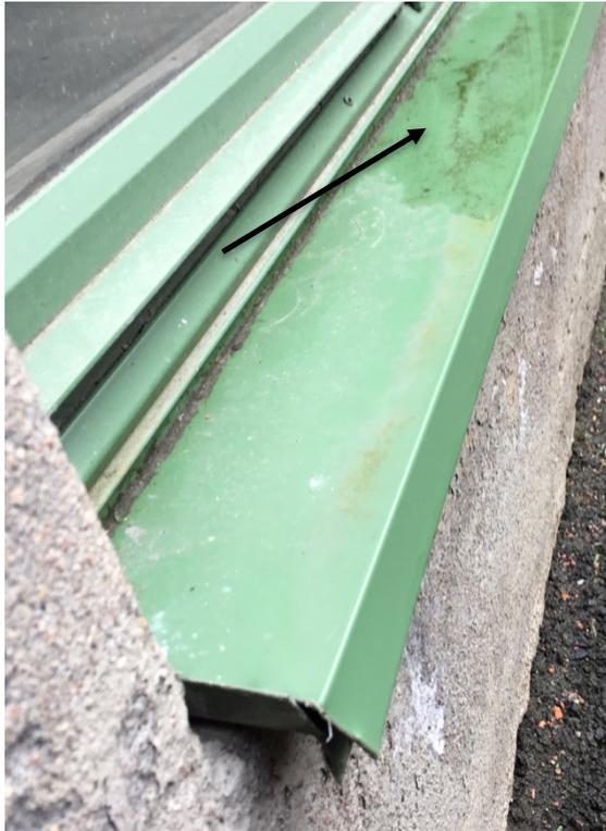
Figure 5.10 Difference in inclination of window ledges resulting in standing water.
