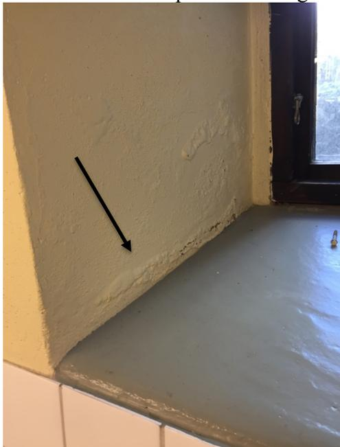
*Figure 5.15 Flaking paint on foundation wall.*
