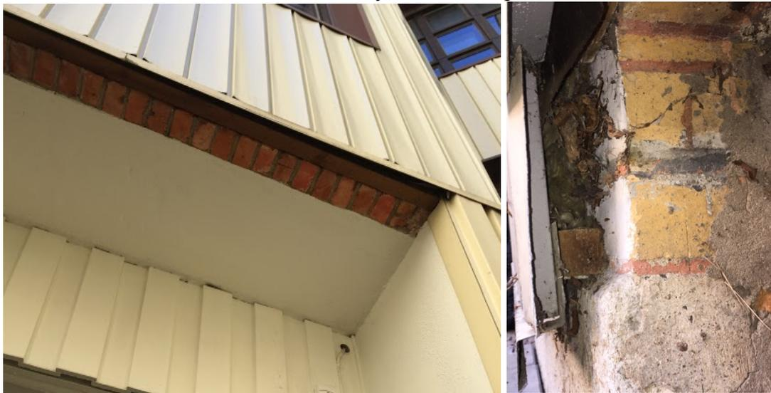
*Figure 5.13 Left: Façade facing to the yard. Right: Added corrugated steel and mineral wool.*
