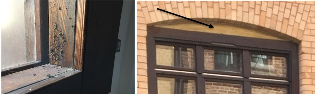
*Figure 5.12 Left: Corner of installed windows. Right: Difference in shape of window and opening in façade.*
