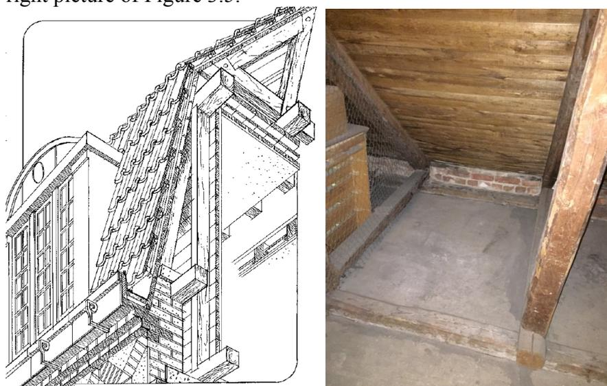
Figure 3.5 Left: Example of connection to wall, mansard roof (Björk et al., 2013). Right: View from the attic of the connection between the external wall and the roof. Notice the brick wall.
