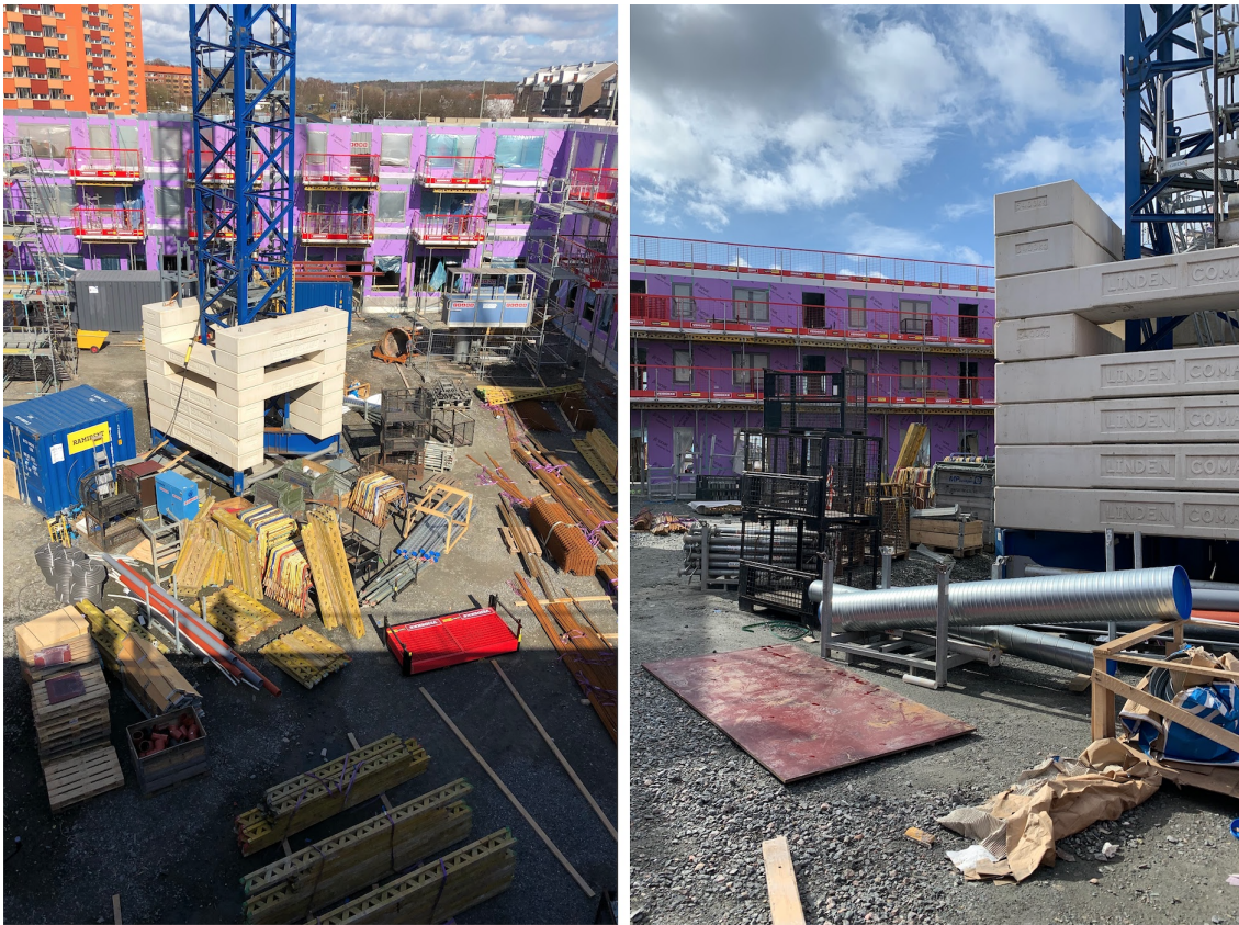
Figure 4.4: Material storage at the construction site.
