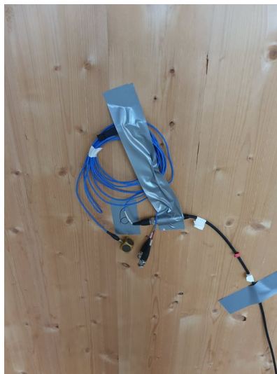
Figure 3.6: Example of a measurement point with cables secured by tapes.
