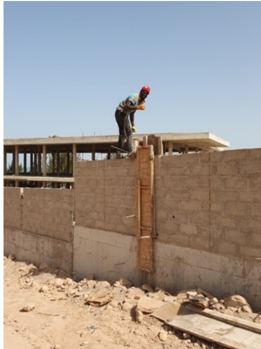
Figure 3.3: Worker on concrete block wall casting a pillar.
