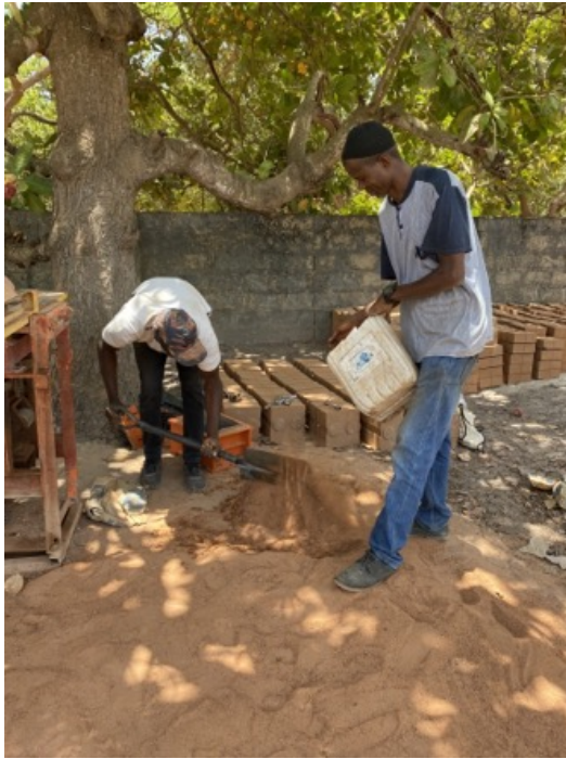
(a) Mixing of earth.
