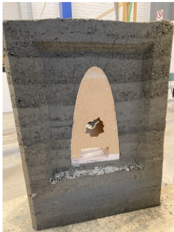
(a) Rammed earth wall with internal arch. The picture is taken just after ramming, with the arch-form still in the wall.
