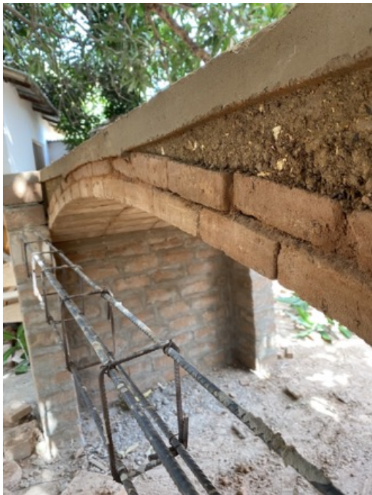
(a) Layers of vault.
