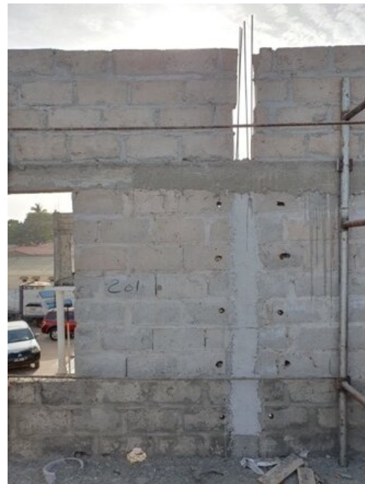
(b) Concrete wall built up with blocks and cast in-situ concrete pillar and beam.
