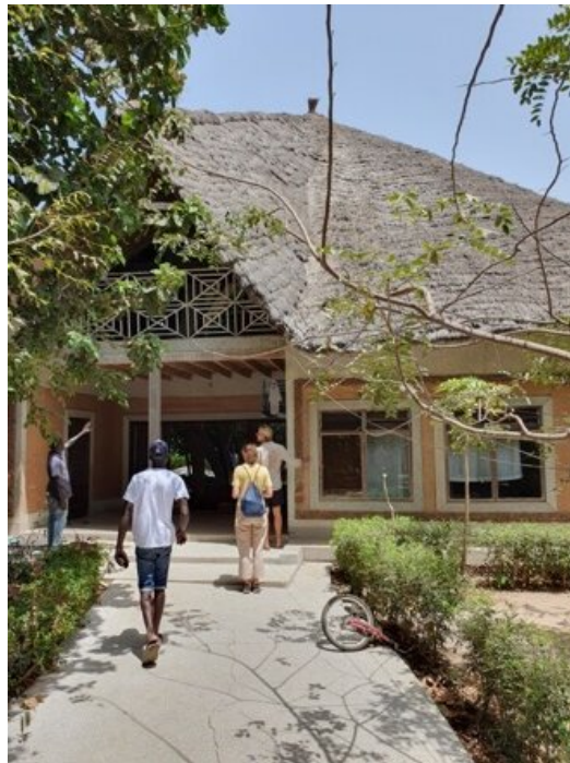
Figure 3.8: Picture of Fake Bachata's house made from CEB with thatched roof and seashell plaster.
