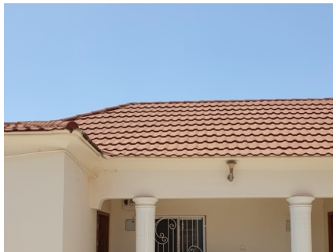
Figure 3.4: Steel roof looking like tiles.
