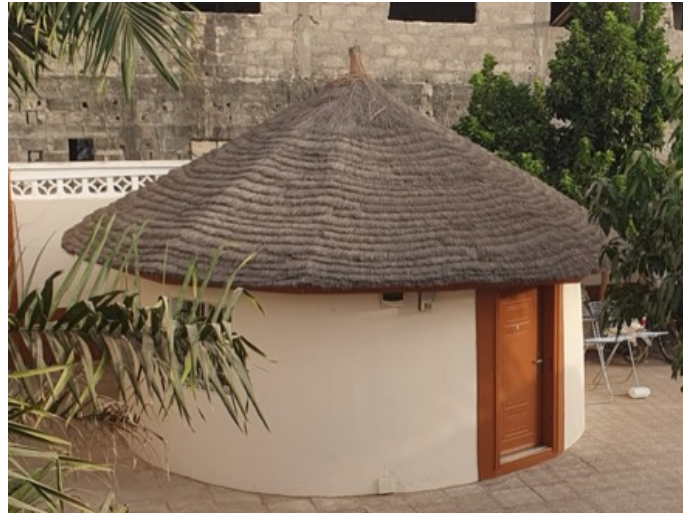
Figure 3.5: Thatched roof with corrugated steel underneath.
