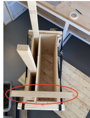
(c) Part of formwork covering the opening.
