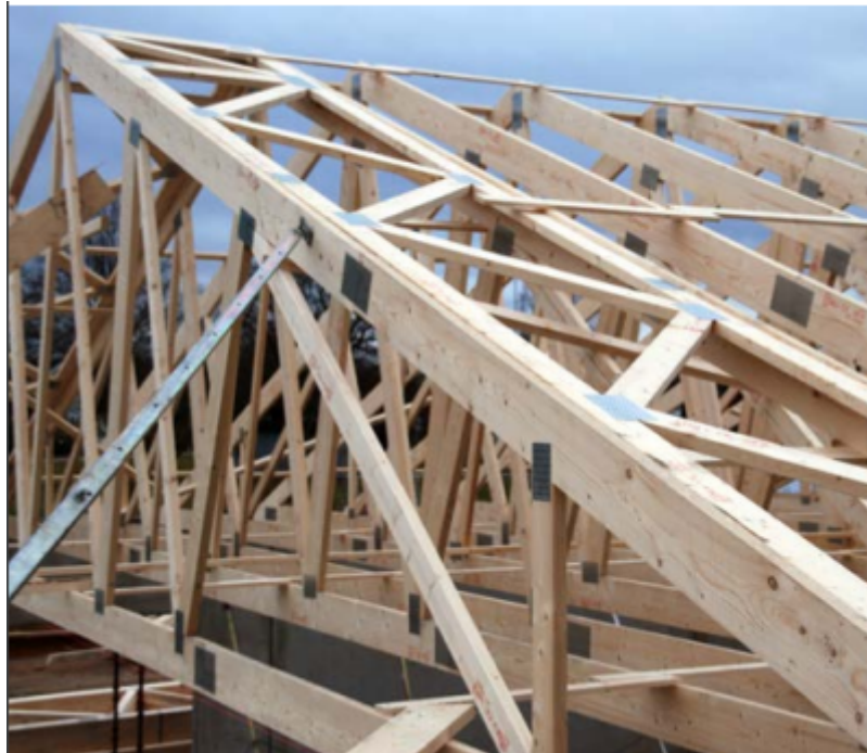
Figure 4.5: Horizontal stabilizing truss for a roof truss, to prevent too large horizontal displacement and failure in that direction (Svenska Takstolsföreningen & Swedish Wood, 2021).
