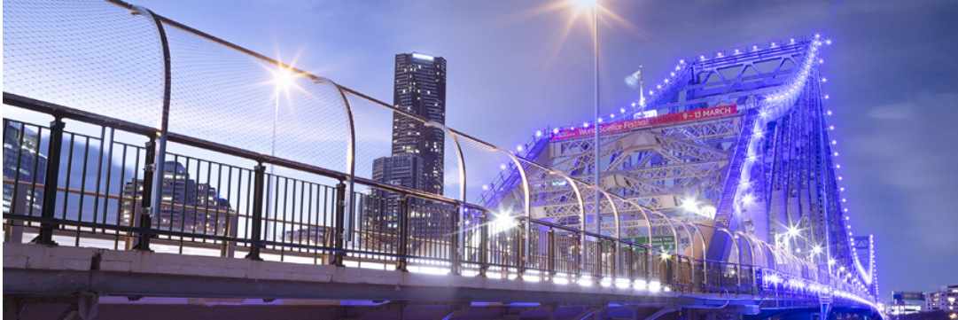
Figure 2.11: Picture of Story bridge, photo courtesy of Atlas steel [5]
