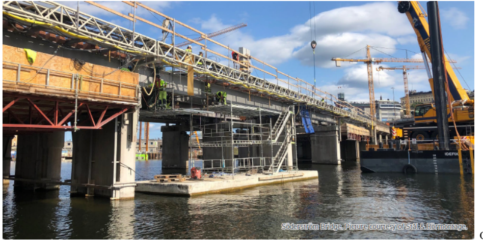
Figure 2.12: Picture of Söderström bridge, photo courtesy of Stål and Rörmontage [4]
