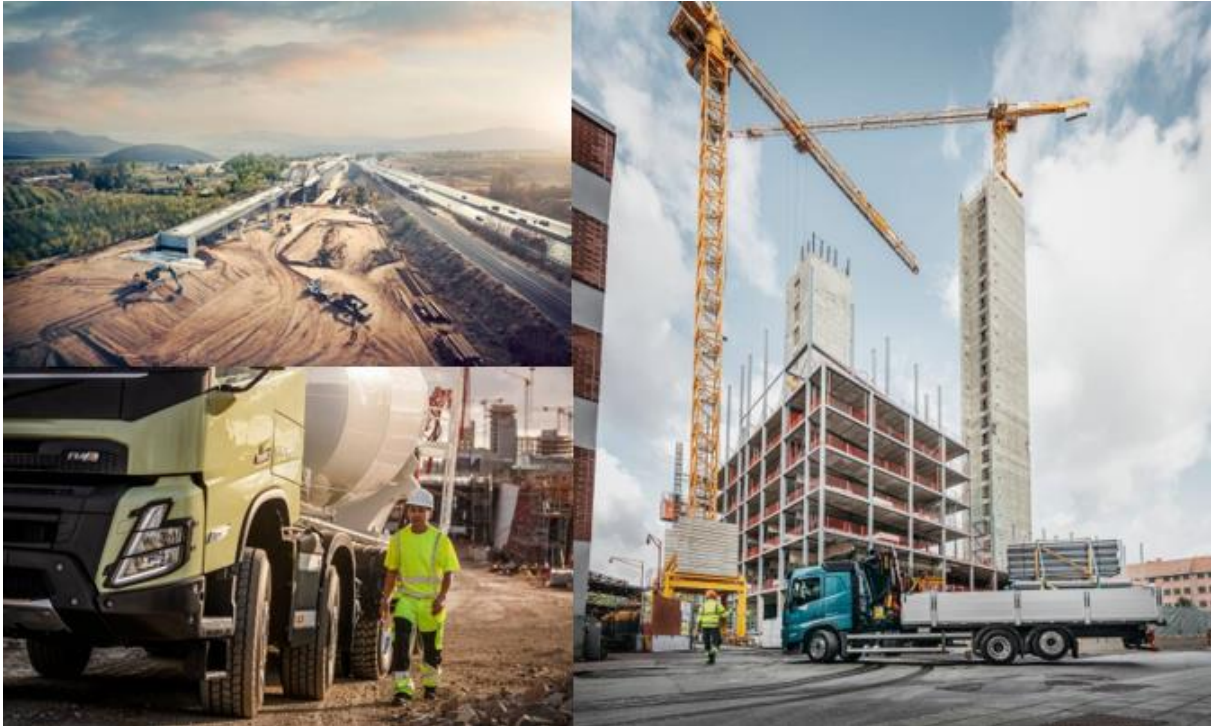
Figure 10. Different construction sites.
