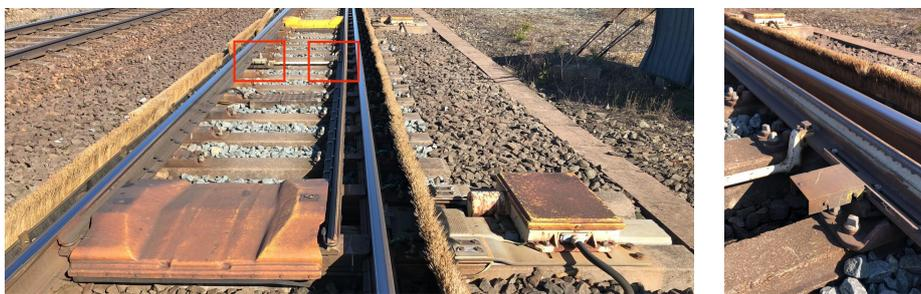
(a) Switching motors with the TKK marked in red. (b) The TKK.
