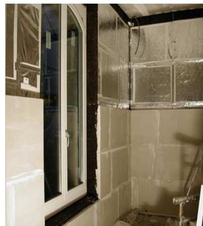
Figure 3.7 Interior Insulation with VIPs in Zürich (Binz et al. 2005)
