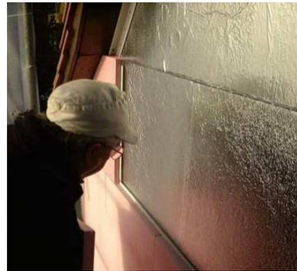
Figure 3.6 VIPs for an external insulation, Germany. On the left, a cross section of the facade. On the right, during the installation (Binz et al. 2005)
