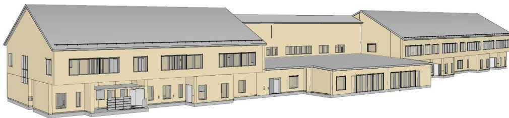
(a) South-west facade.
