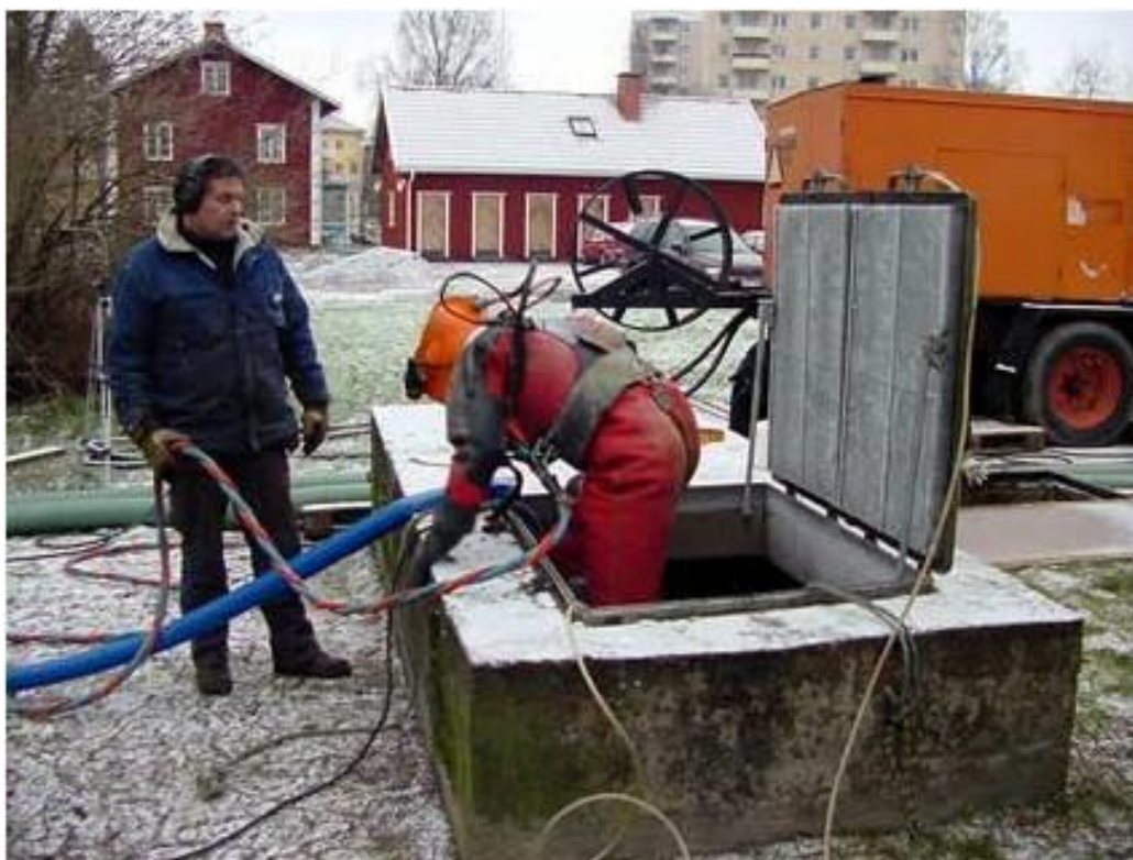
Figure 3.3.3 A diver is on his way down to repair the overflow function to stop the water at Landa pumping station (Kristinehamn municipality)
