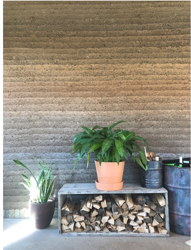
Illustration 27. Image rammed earth wall. Photo: Klara Moene-Omholt
