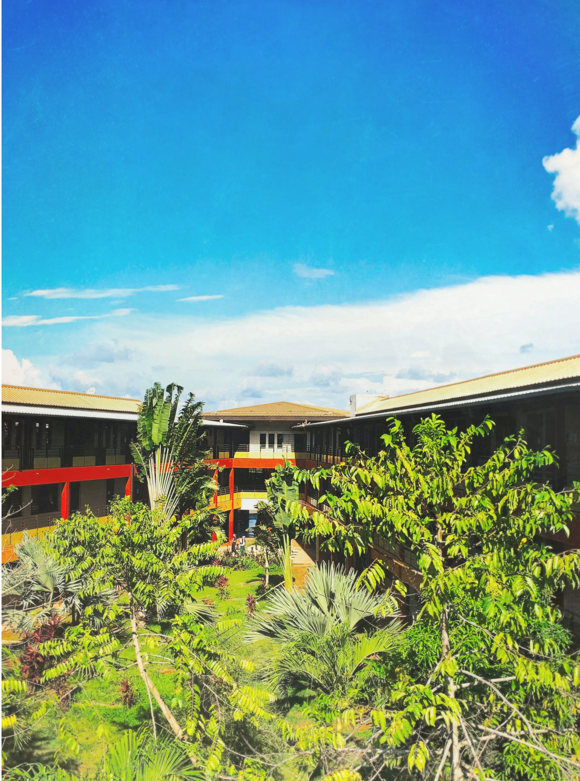
figure 5.1 : View from the yard, High School "LYCÉE DES LUMIÈRES", Mamoudzou, Mayotte
