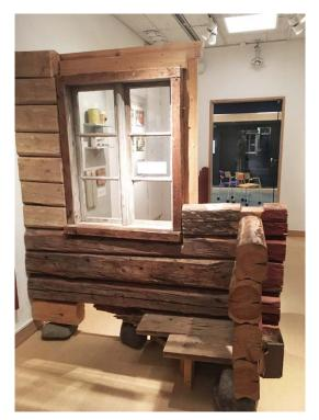
Figure 15. A timber wall without panelling.
