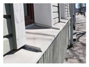
Figure 71. Sill of a window that rests on a level-ribbon.
