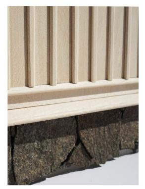
*Figure 121.* Panelling meets the foundation. Original scale 1:10.
