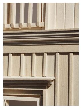
*Figure 123.* Head casing, level ribbon and railing of the french balcony. Different depths of the facade. Original scale 1:10.
