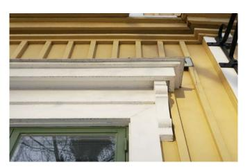
Figure 49. Head casing of a window.
