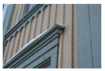
Figure 53. The headcasing of the window on the first floor.
