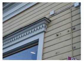
Figure 60. Head casing of a store window.
