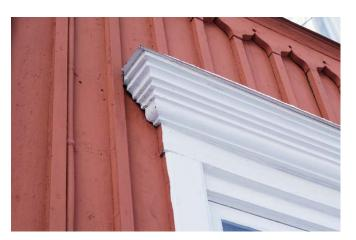
*Figure 43.* The head casing of a window.
