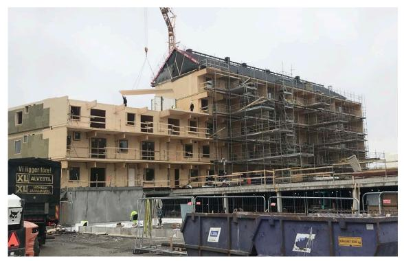
Figure 2. Construction of a multiresidental building in cross laminated timber, Växjö.
