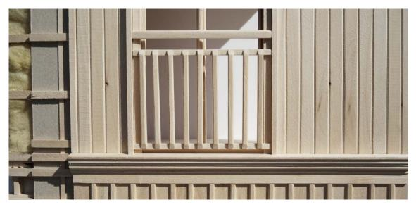
Figure 120. Zoom-in of a french balcony railing and the level ribbon. Original scale 1:10.
