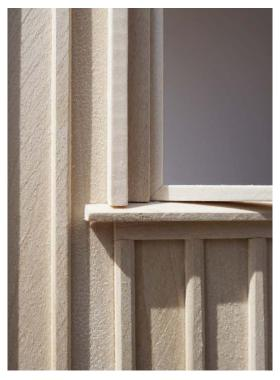
*Figure 122.* Window sill and side casing at entrance floor. Original scale 1:10.
