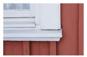
*Figure 44.* The sill of a window.
