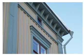
Figure 56. Facade, showing the depths of the panels.
