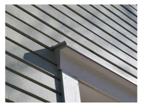
*Figure 70.* Head casing of a window.
