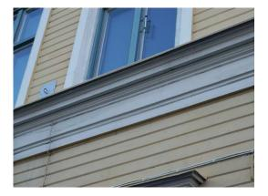
Figure 61. Big, profiled batten separating the floors.
