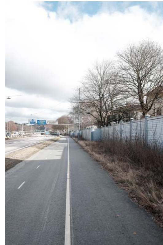
The sound barrier turns into a board along the entire block of Törnrosen and separates the houses from the traffic route, as well as
