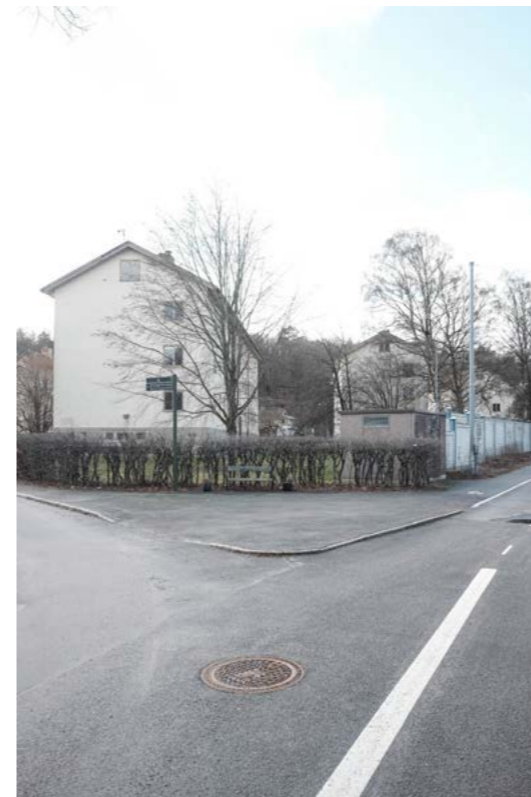
The opening in the sound barrier is right at the beginning of Kv Törnrosen. Here you meet the short sides of the slats, which are separated by a
