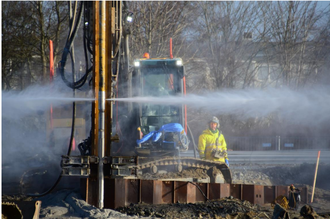
Figure 32 The jet stream using two nozzles. Note that here only water is flushed through the system.
