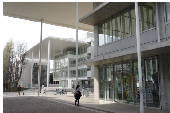
Picture 18. KOMCEE building. Authors' picture.
