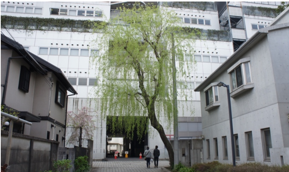
Picture 21. Komaba 2 East entrance. Authors' picture.
