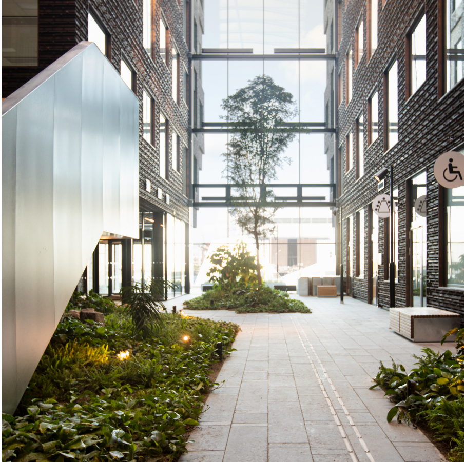
Figure 4.2: The green atrium of Epic, with reused wood as the wooden panels (Skanska Sverige, n.d.).
