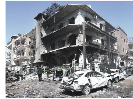
Image 05: One of the bombed buildings
