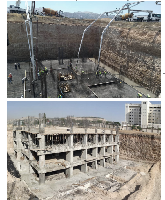
Images 18,19: Marota city construction [Top-down]
