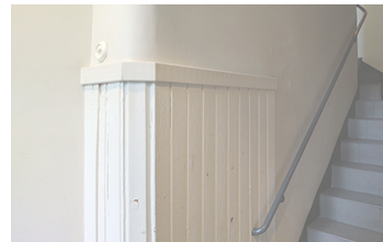
4. Details 1891, original staircase situation
