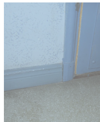
9. Door and wooden details, 1926
