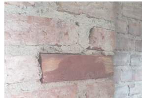
6. Old cracked brick firewall, repaired with wooden bricks
