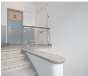
8. Stairs with granite details, 1926
