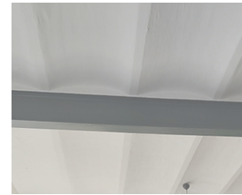
1. Molded vaults, Beams structure and pelars from 1898
