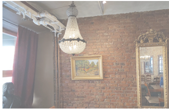
1. Bearing wall in bricks from 1891
