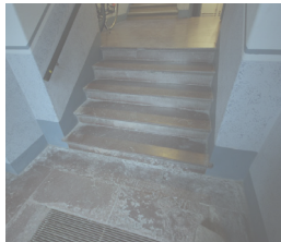
5. Original staircase from 1926
