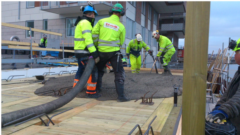
Figure 3.25: Casting of the concrete slab during the construction of the quay. Some of the rebars that are soon to be cast into the concrete are visible. (ÅF, 2015)
