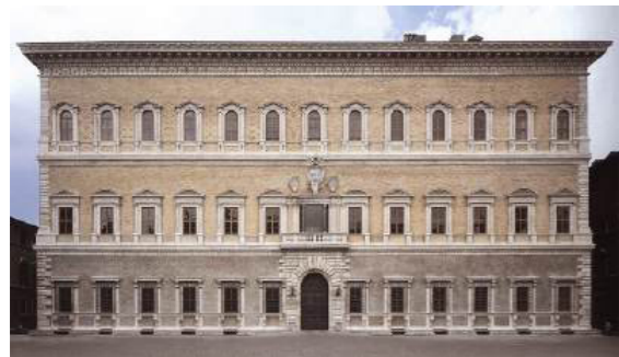
Fig.13: Michelangelo skillfully added a floor to the Palazzo Farnese, originally designed by Sangallo the Younger, redefining the proportions and visual focus of the façade with a delicate touch.
