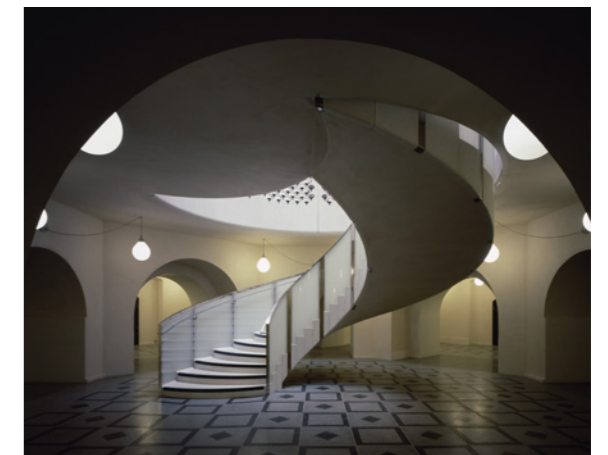
Fig.15: For the Tate Britain at Millbank, they enhanced and renovated the rotunda at the Millbank entrance by drawing on the original design's ceremonial qualities, materiality, and proportions, introducing a new spiral staircase that enriches the spatial experience.
