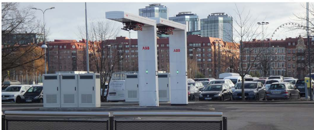
The bus ring and charging stations in between Heden Bus Terminal and Exercishuset
