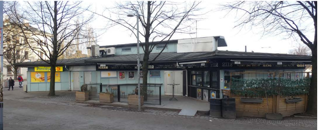
Existing Heden Bus Terminal, viewed from west
