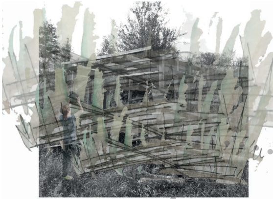
Image 75.2 Art hall : collapsed & overgrown.
