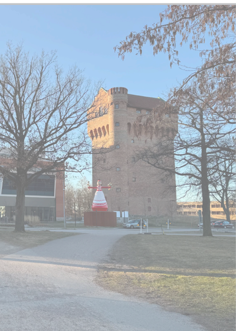
View towards CV Water tower
