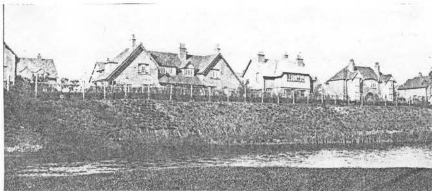
Bournville. Backs along Elm Road.
