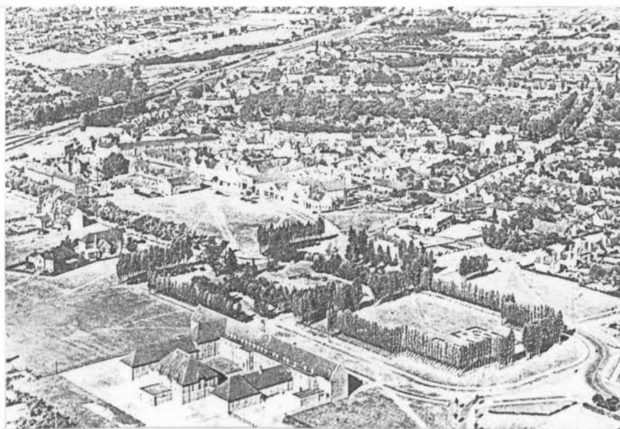
Letchworth, Aerial view of the centre 1930-35.
