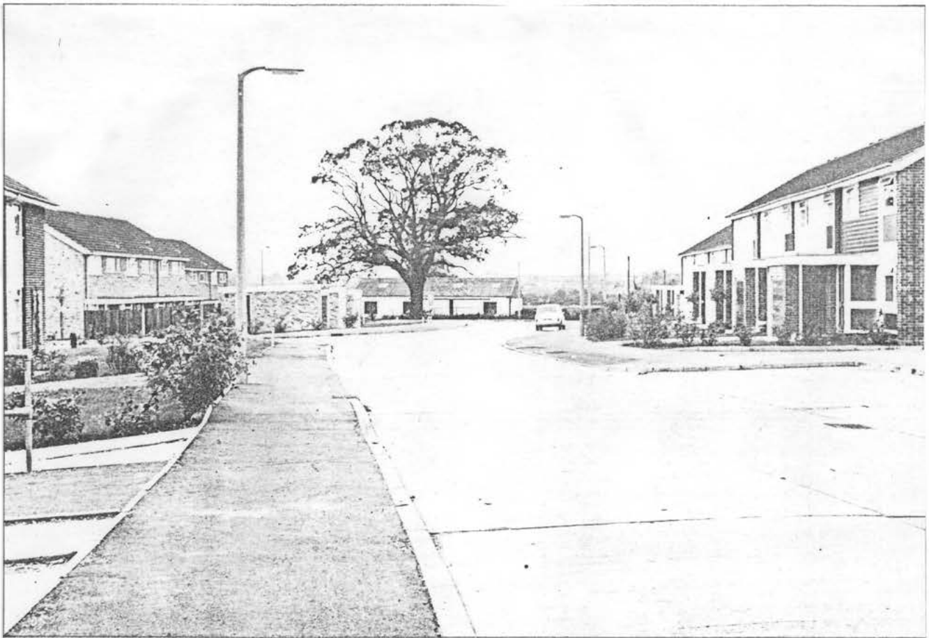
Typical Suburban Scheme in England where regulation street and pavement widths gave rise to what became known as "Prairie Planning".
