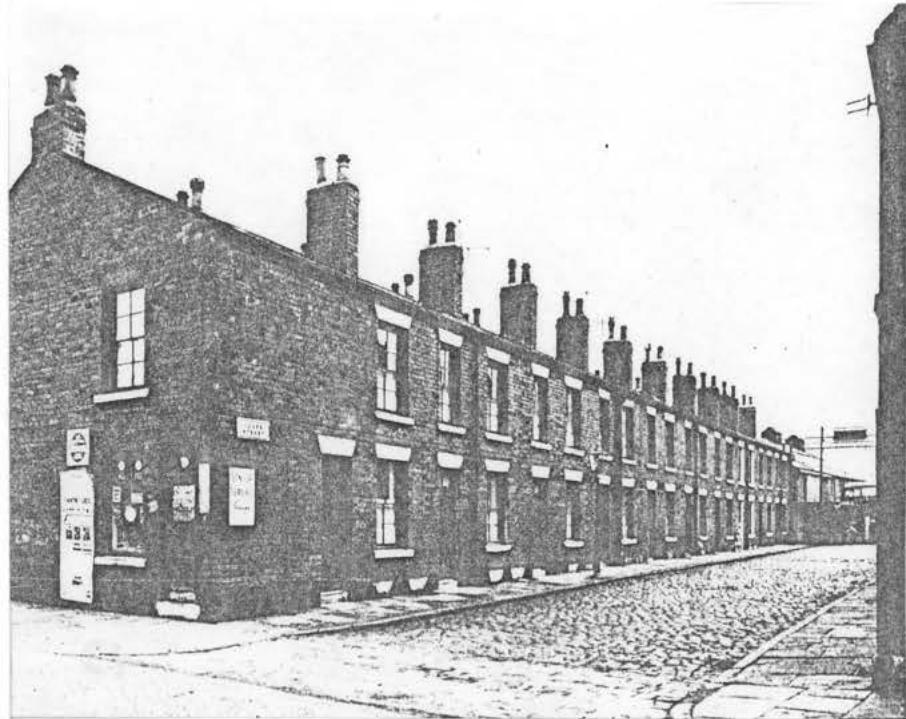
Clark Street, Saynor Lane, Hunslet District, Leeds. 1850-60. Back to back housing. One room downstairs, two upstairs. Sanitary conveniences at the end of the row.
