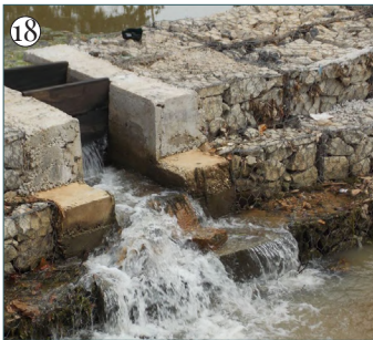
Gabion check dam
