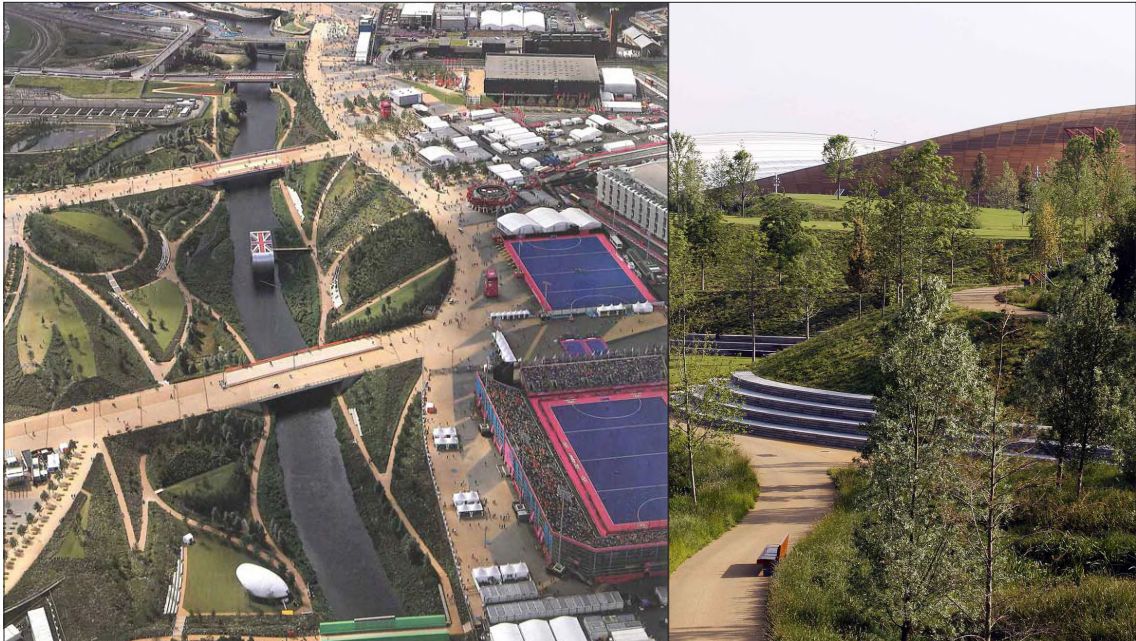
Figure 2.14. Queen Elizabeth Olympic Park demonstrates how urban land can be transformed into resilient green infrastructure through sustainable resource management. Source: Hargreaves Associates. (2016, July 28)
