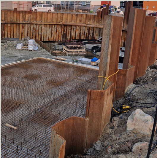
Figure 2.09. Reused sheet piling. Photo by the author.
