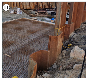
⑪ Reused sheet piling
