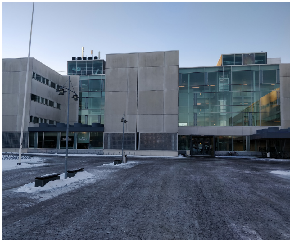
Eastern and southern facades of buildings around my site (facing the square)
