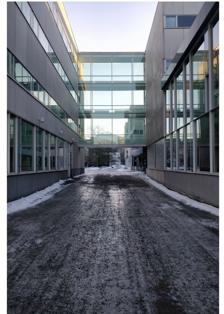
The room between the existing buildings
