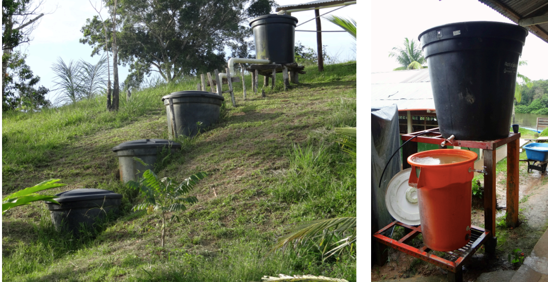
Picture 1.1. Left: The three-step system built 2006 by Andersson and Erlandsson. Right: A two-step system next to the school in Puerto Rico.
