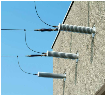
Figure 2.2: Air to Air - Wall Bushing [19]
