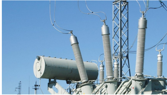
Figure 2.1: Air to Oil - Transformer Bushing [18]
