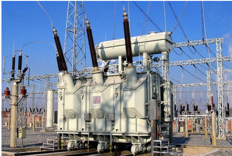
Figure 1.1: Power Transformer [1]
