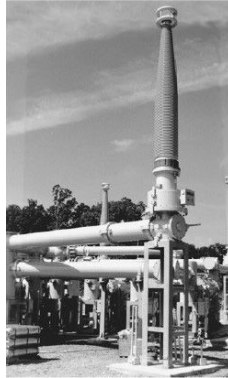
Figure 2.3: Air to SF 6 bushing [20]
