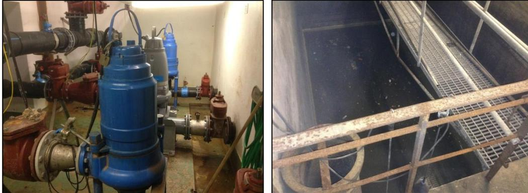
Figure 14 To the left; dry sewage pumps and to the right; separate sewage basin
