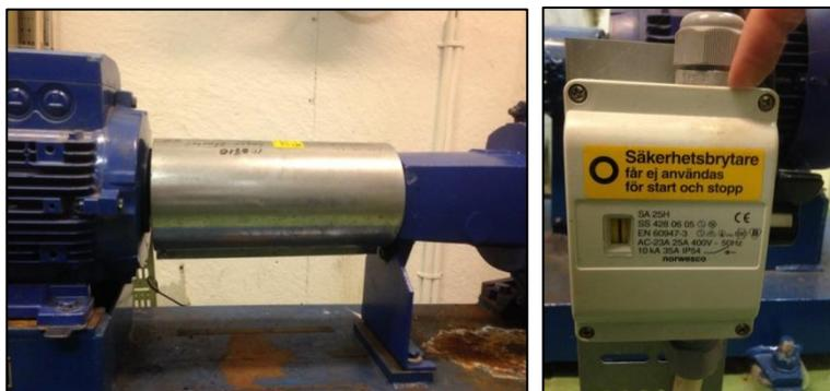
Figure 10 To the left; pumping shaft on a drinking water pump and to the right; security power switch
