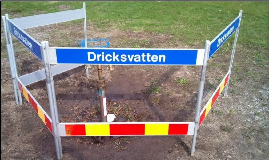
Figure 18 Temporary station for drinking water distribution from fire hydrant
