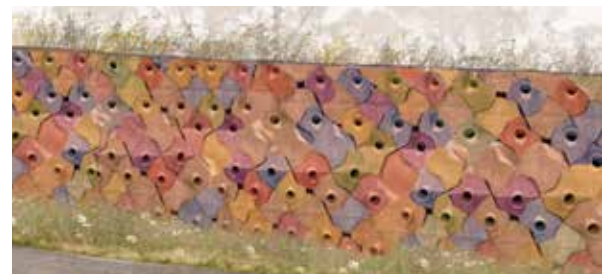
Section of the Helmholtz resonator wall
