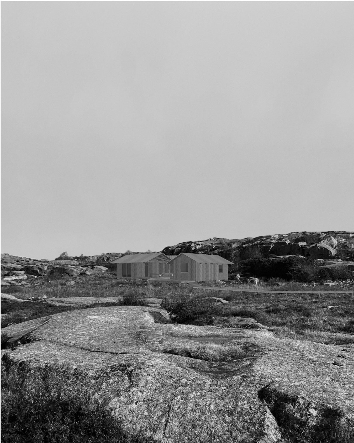
View of service facility from the southeast.
