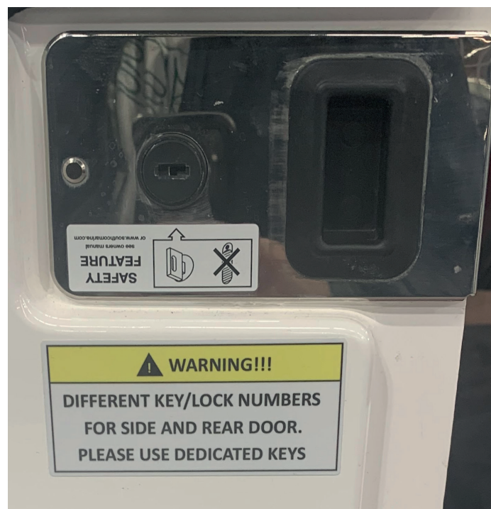
Figure 13: Note on boat cabin door reminding user to keep track of keys.
