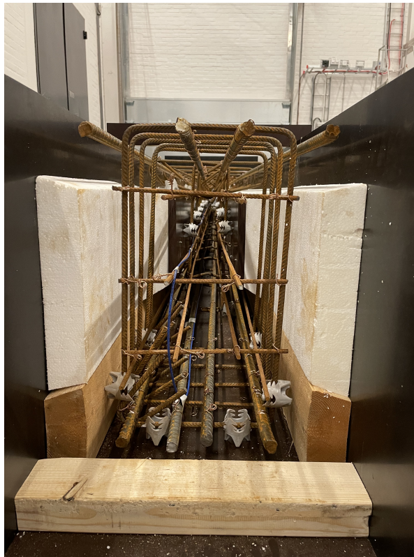
Figure 4.3: Reinforcement in formwork.
