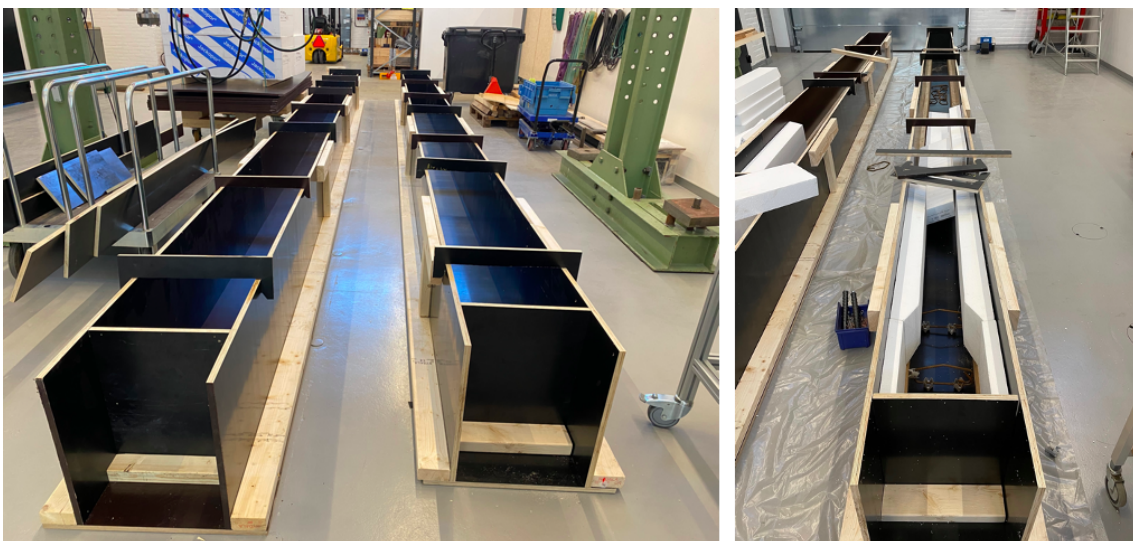
Figure 4.2: Construction of formwork.
