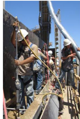
Figure 15 Modern earth ramming, (Photo by David Easton, n.d.) →
